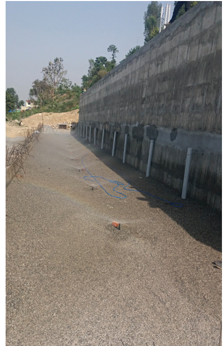
Sewerage Treatment Plant
